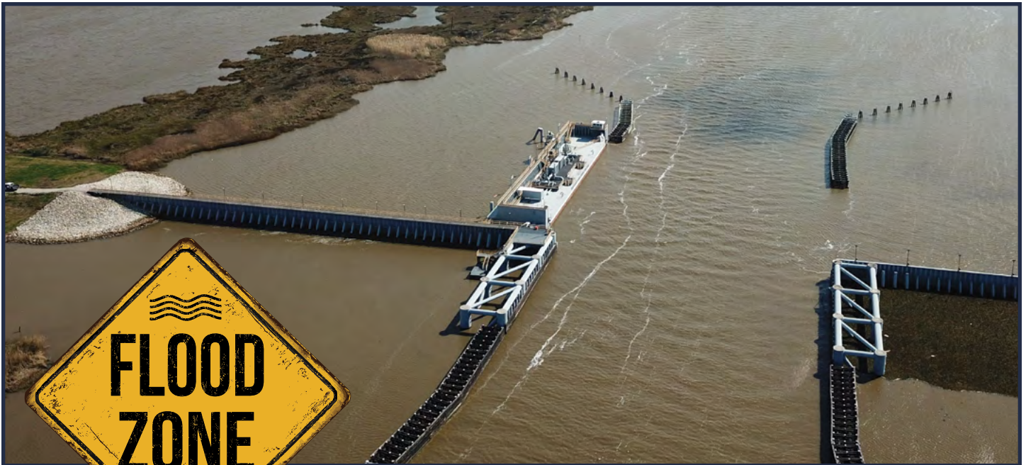
Local initiative and ingenuity are protecting Terrebonne Parish, Louisiana, from storm surges. Since 2007, $414 million has been invested on flood protection in region; locals have paid 57% of the tab.
